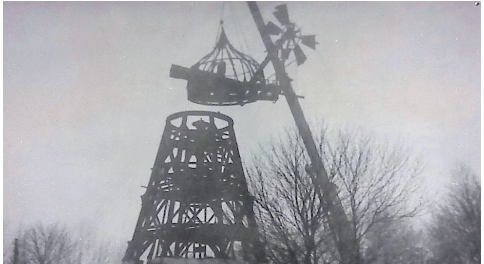
Crane lifting cap off of the mill
