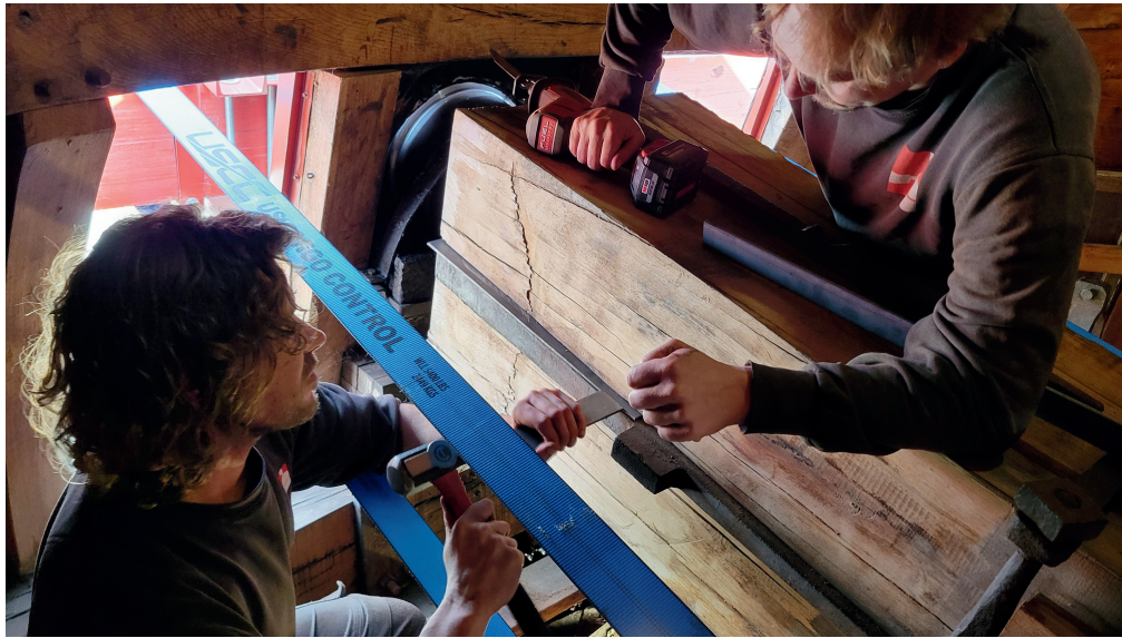
Erik and Ronald hammering the steel shims into the windshaft.
