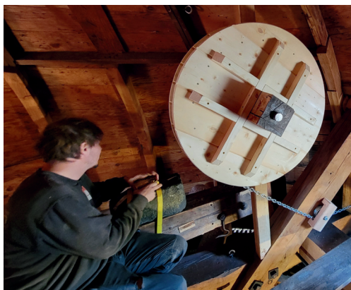
Erik finishing the new wheel and axle for the brake pulley
