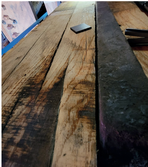
The gap between the windshaft's oak and cast iron
