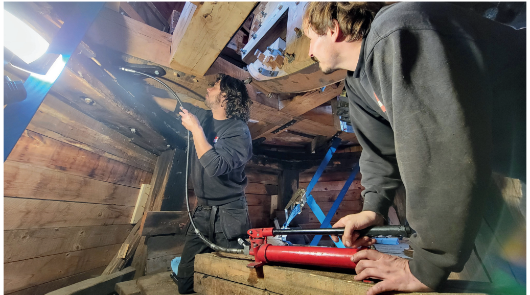
Ronald & Erik using a hydraulic jack to lift a contact point on the cap frame
