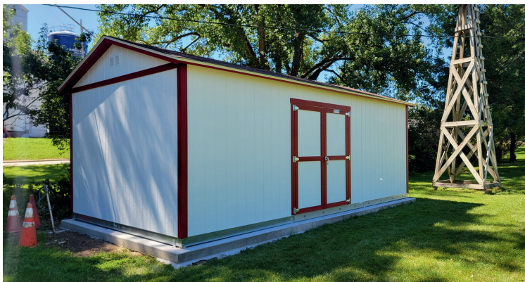
Our new entertainment & storage building
