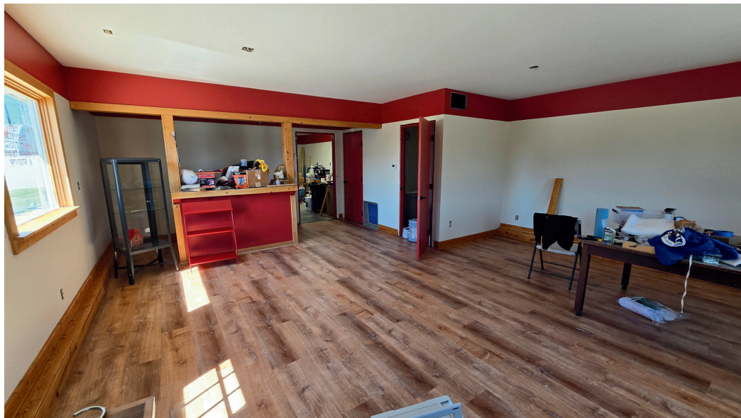
Work on the classroom side of the PEC is underway
