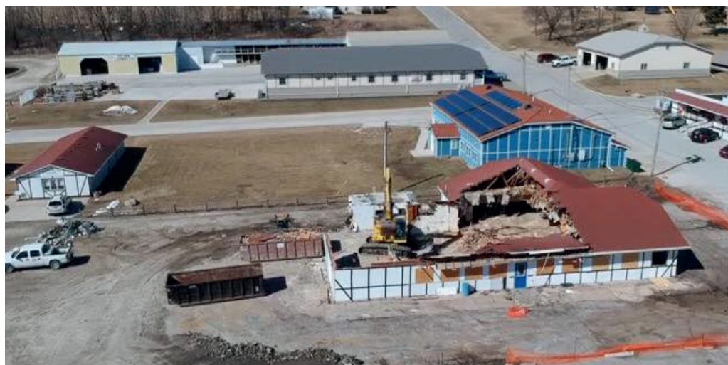
The Danish Inn during demolition in 2018 with the new building (blue) behind it
