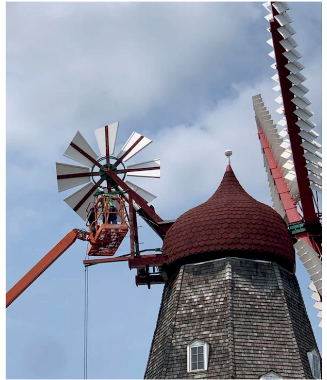
Shaun Sayres & Tim Palmer working on the fantail Photo by Brandon Baggett
